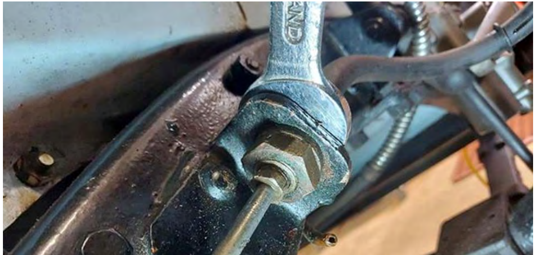
Removing brake line and flexible hose from the frame bracket using the CORRECT sized Whitworth spanner.
